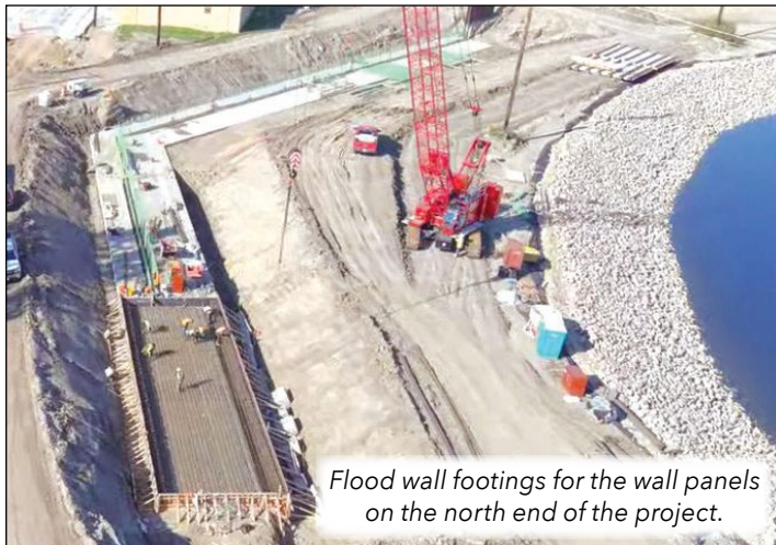
Trenching machine for the flood wall footings.
