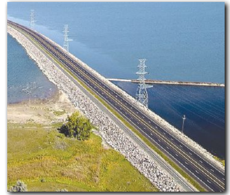
Snake Creek Embankment
