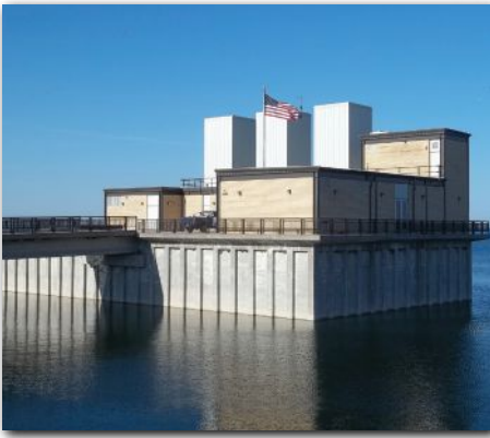
Snake Creek Pumping Plant
